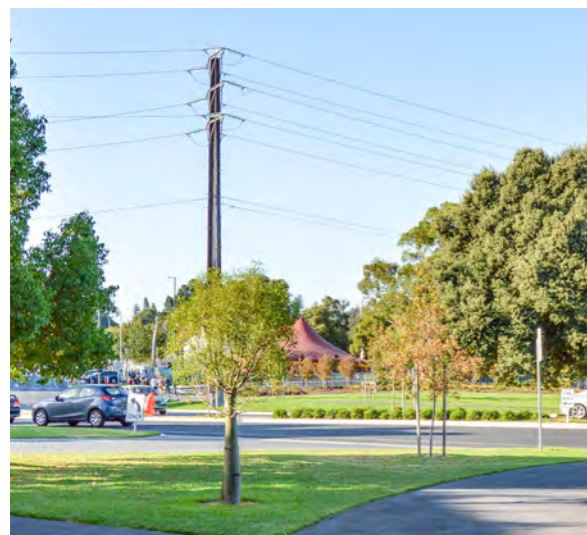
Existing Stobie poles dominating the Park
